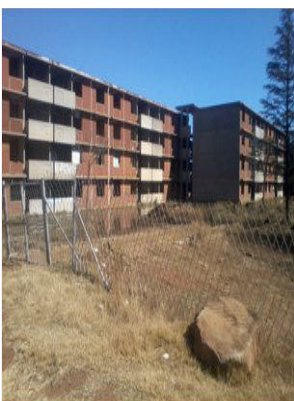
The old Kwa Masiza hostel, going under refurbishment.
